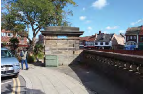
The Old Town Bridge Pier
