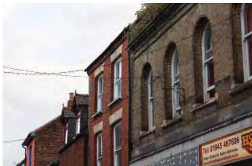
Windows at first floor level
