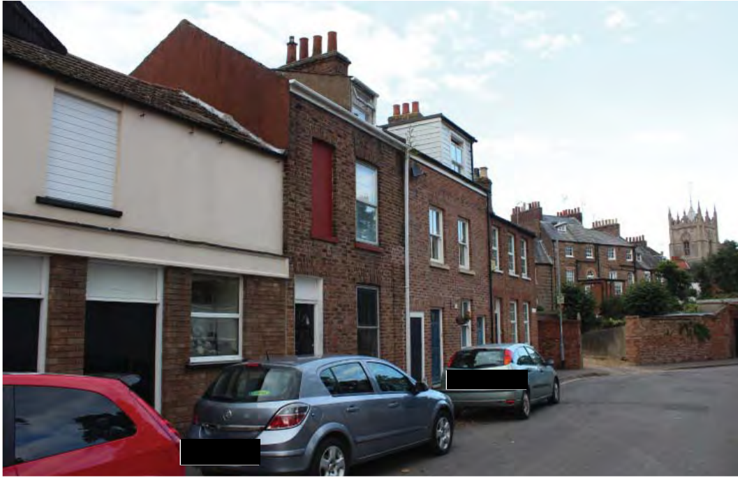
Buildings along Love Lane has suffered from a number of inappropriate alterations which detract from the historic character of the buildings
