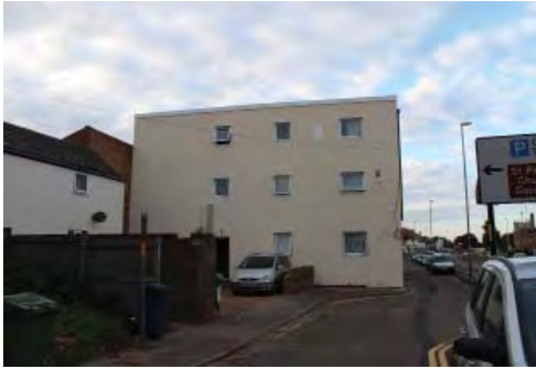
View looking north along Churchill Road. This building, clad in external insulation, does not contribute positively to the area
