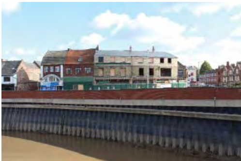
1 Nene Quay, in the process of restoration.
