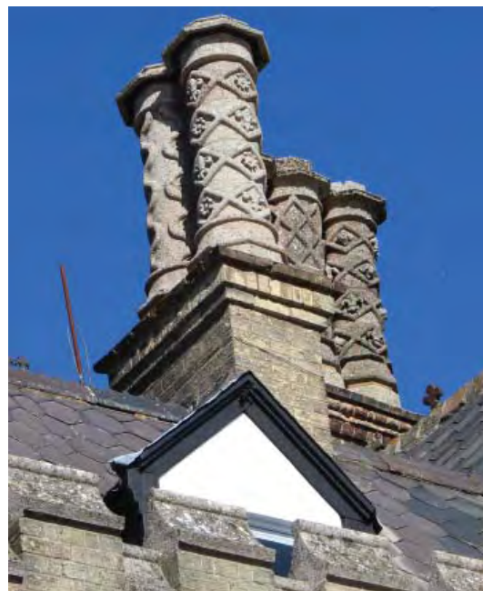
Elaborate chimney stacks on Nos.23-24
