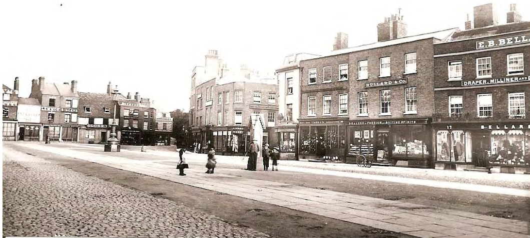
The Market Place in the mid-nineteenth century, illustrating the quality and character of the shop frontages in the area at that time
